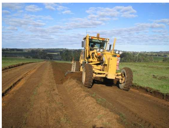
Plate 2. A road grader mounds soil into a treeline bank
