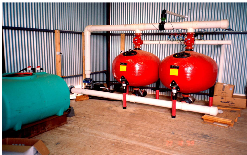
Plate 5. Fertigation tank (LHS) and irrigation filters (RHS)
